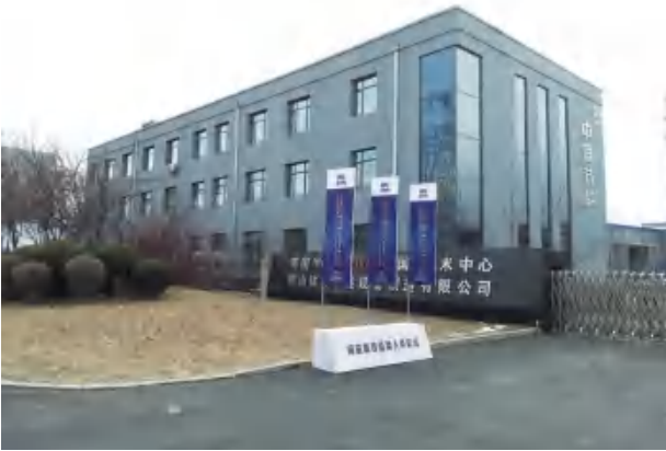
Fig.6 Picture of Magna Project Plant Area
