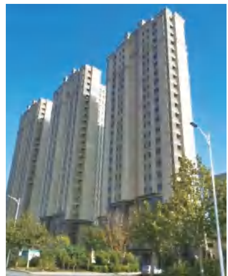
Fig.2 Picture of Hutchison Whampoa Project in Dalian
