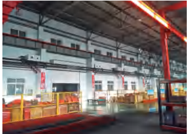
Fig.7 Picture Inside of the Plant Area of Magna Project
