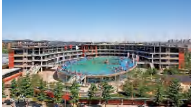
Fig. 21 Wanliu Area Primary and Secondary School Joint Project Scene
