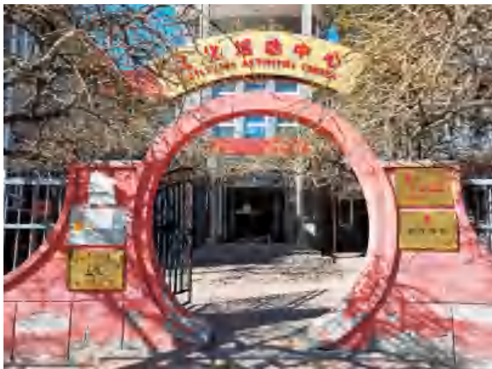
Village cultural center heated by ground energy heat pump
