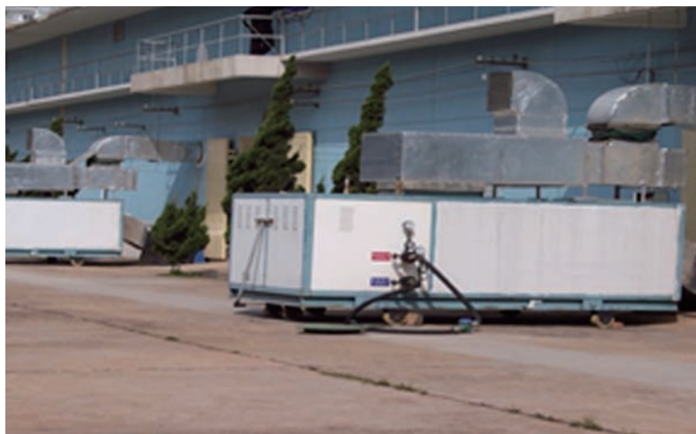
Ever Source's Single Well Cyclic Heat Transfer Geothermal Energy Collection Well and Mobile Heat Pump Device
