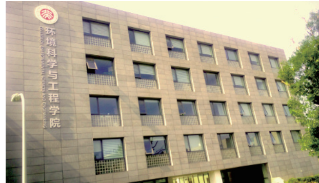
Building of College of Environmental Sciences and Engineering
