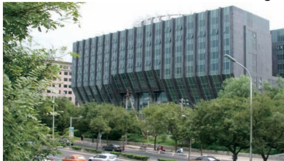
Office Building of All China Federation of Industry and Commerce: 50,000m 2
